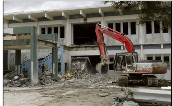
Whitaker being demolished in 2007
